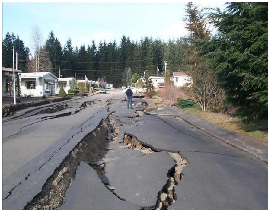
(Figure 46: soil liquefaction)
